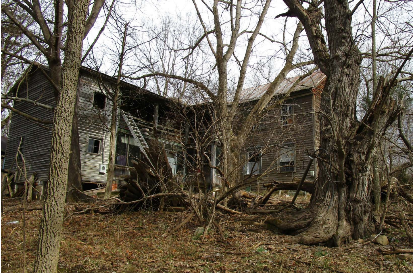
View from the back side of the house where the newer “ell” addition is visible on the left, and the original part of the house is on the right. If you peek under the clap board, the original logs can be seen. Photo by Marie Rasnick Fetzer.
